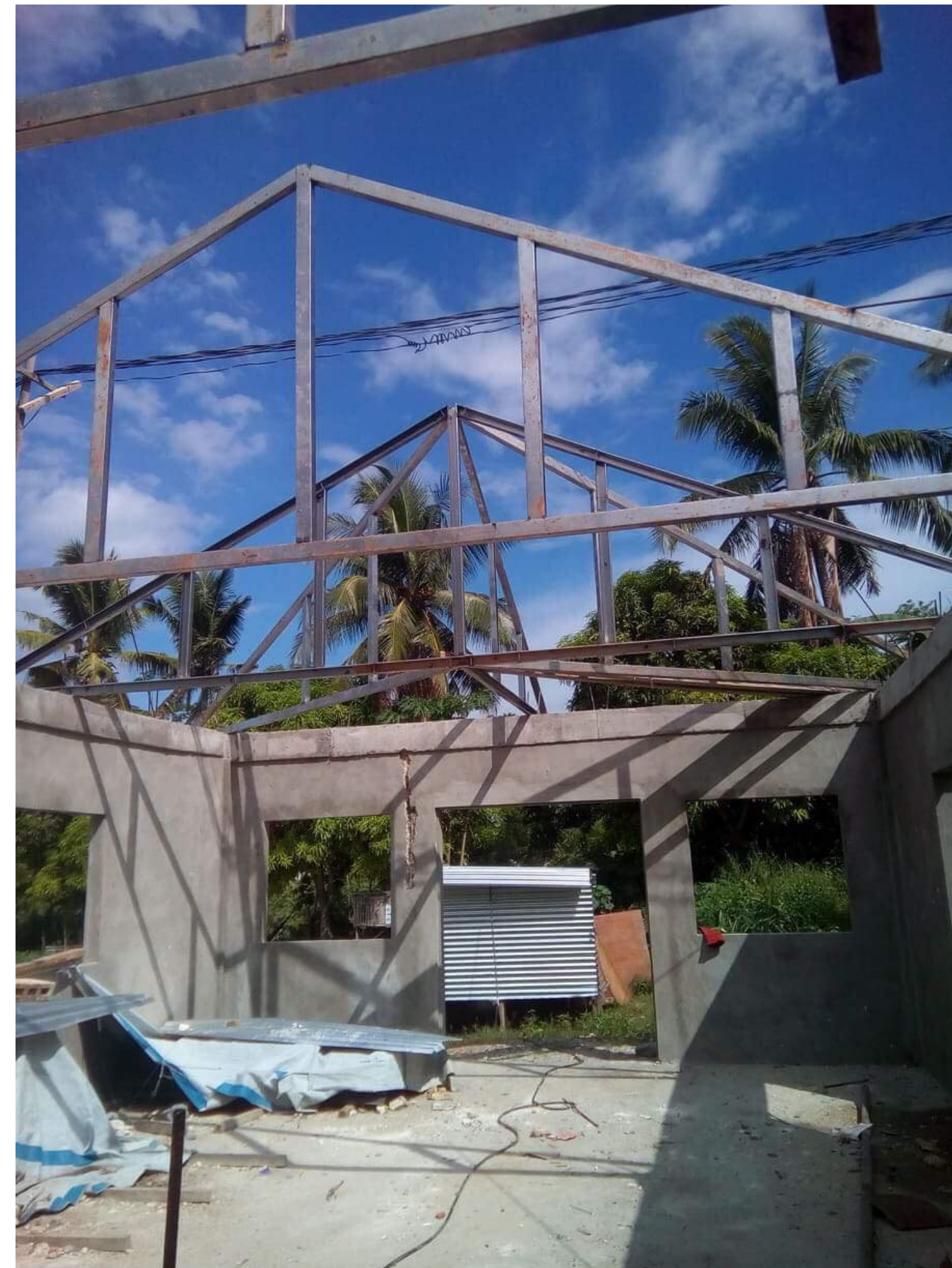
Installation of roof trusses, June 2018
